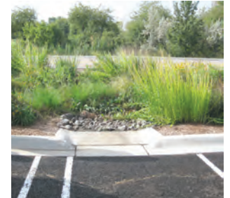
Figure 55: Parking lot bioswale precedent
