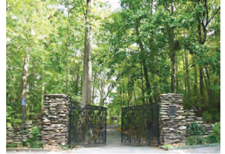
1. Nevada Avenue entrance gate (Figure 46)
