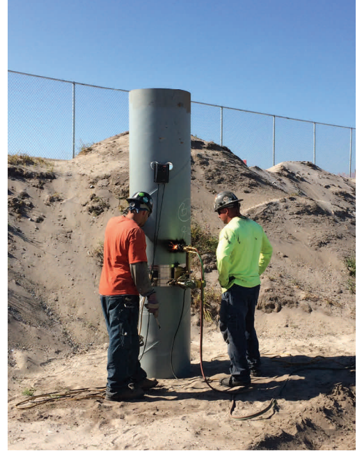
Phase 1— Pipe Pile cutting
