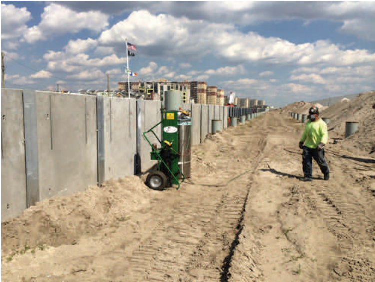
Phase 1 — Sand retaining wall installation (beach side)
