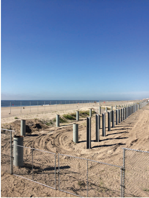
Phase 1— Pipe Piles and H-Piles
