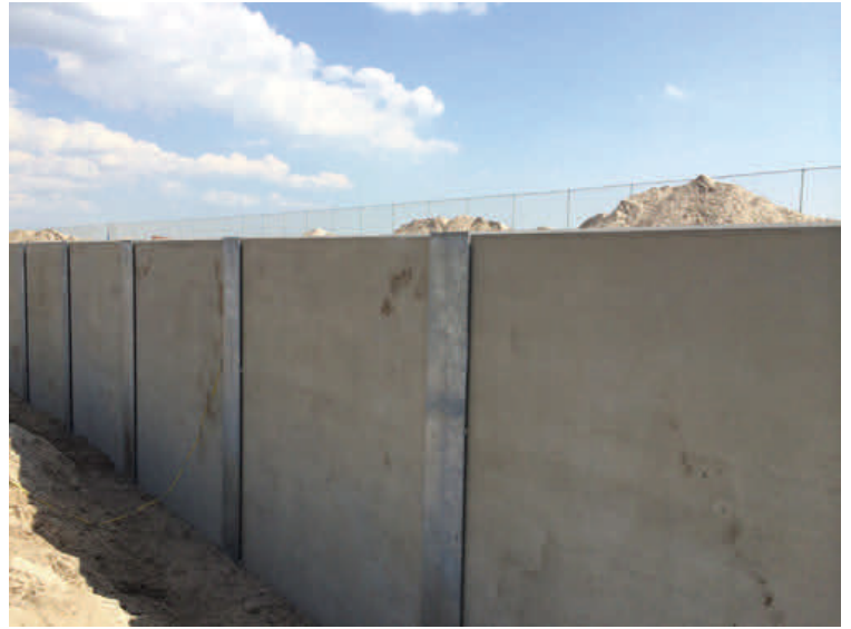
Phase 1 — Sand retaining wall installation (land side)
