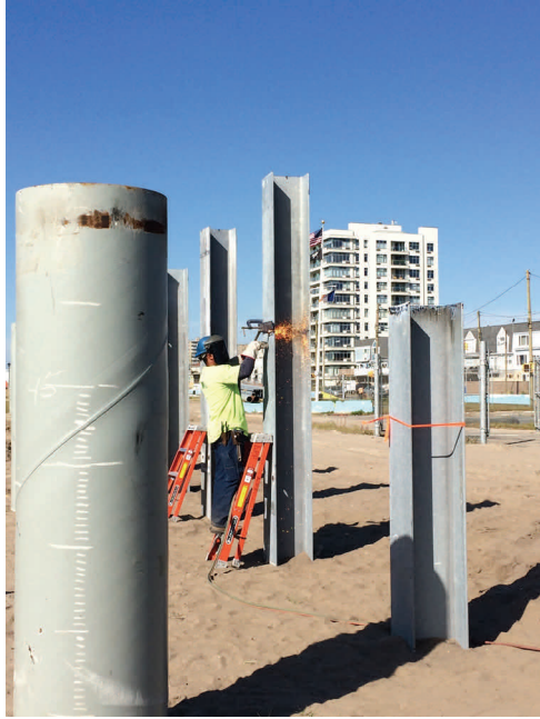
Phase 1—H-Pile cutting
