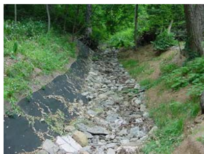
5) Partially Restored Gully in Inwood Hill Park
