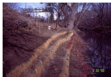
11) Coirlogs and live stakes installed behind Metro-North Woodlawn station platform
