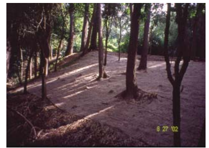
3) Jute mat on hillside at Riverdale Park, prior to planting
