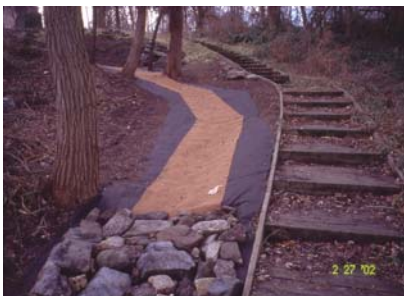
7) Work in progress on a gully at Seton Falls Park.
