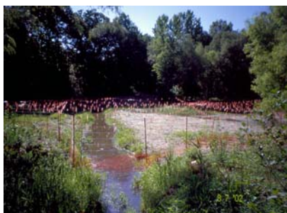
4) Recently planted wetland at capital project site in Seton Falls
