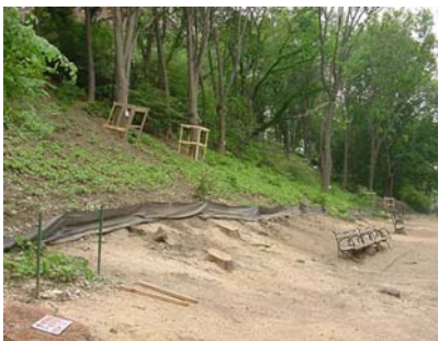
1) Riverside Park under construction
