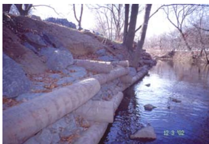
10) Log crib structure at 226th Street on Bronx River
