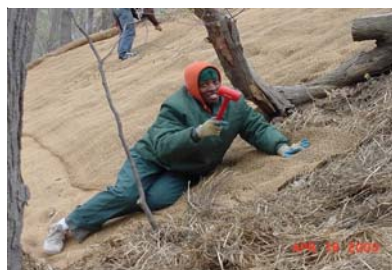
17) POP participant installing erosion fabric
