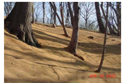
3) Slope stabilization at Riverdale Park
