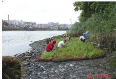
9) Installing coir mats at the Lafayette Ave. site
