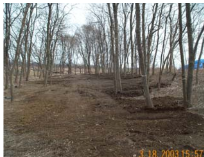
During capital construction
