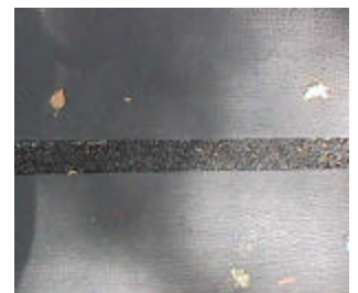
Filled safety surface gap
