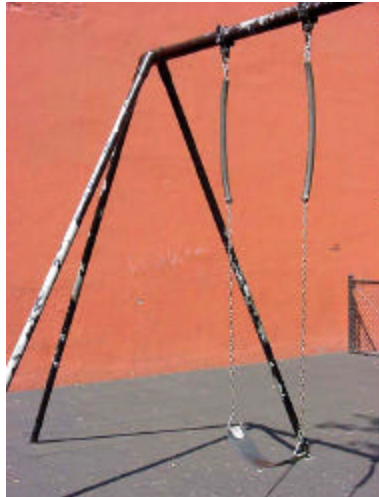
Rubber hose protects swing chains
