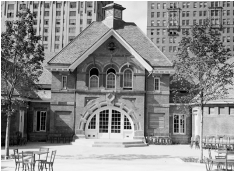
Arch construction before and after, 1934.
