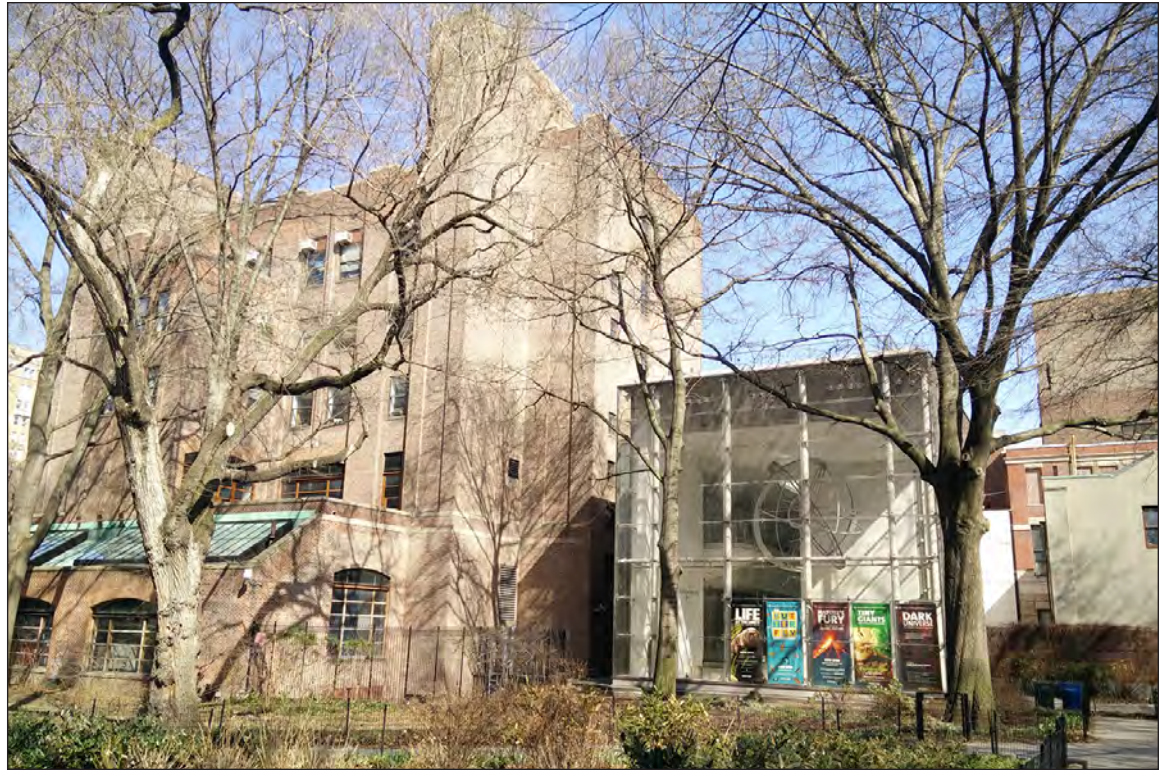
View of Existing Building 17 and Weston Pavilion 5
