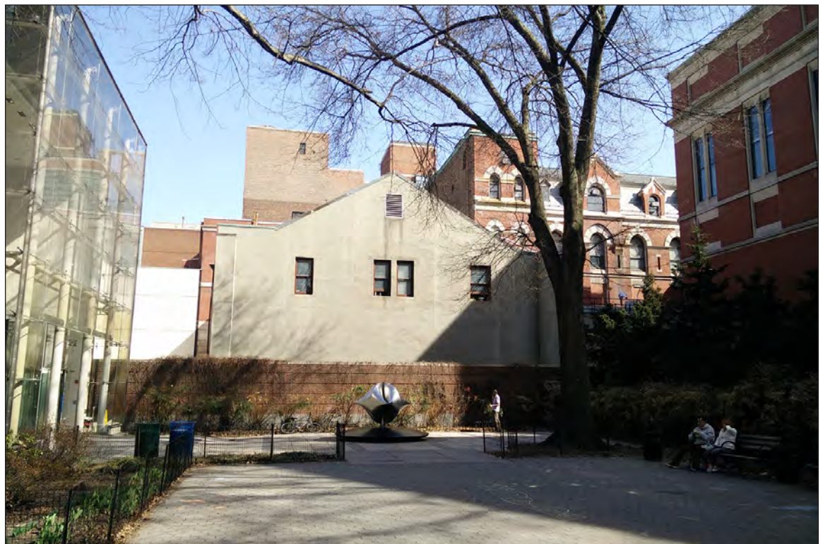
View of The New York Times Capsule and Building 15 Facing East within Theodore Roosevelt Park 6
