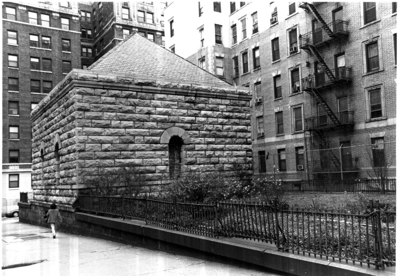
Croton Aqueduct West 119 th Street Gatehouse Upper: entrance Lower: south elevation and grounds Photos: Carl Forster
