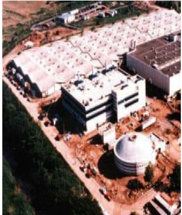
Figure 8: Oakwood Beach Treatment Plant, Mill Road
