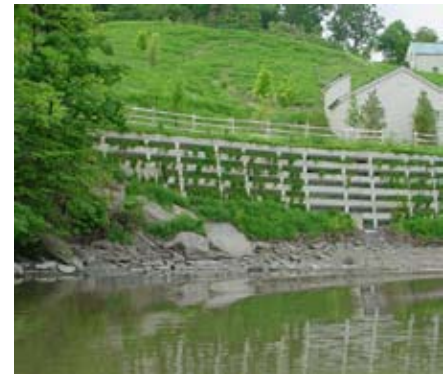
“Evergreen” Greenwall, near Athens, NY. Photo: LI Precast
